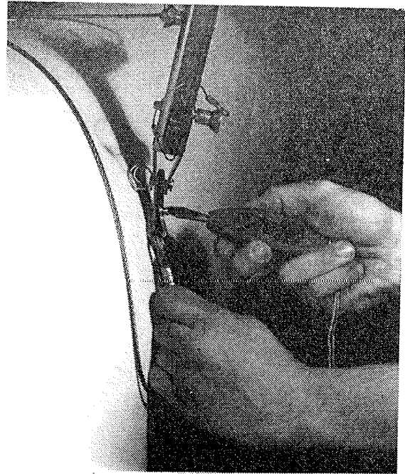
Photo F4. Installing the shroud extension assembly.
